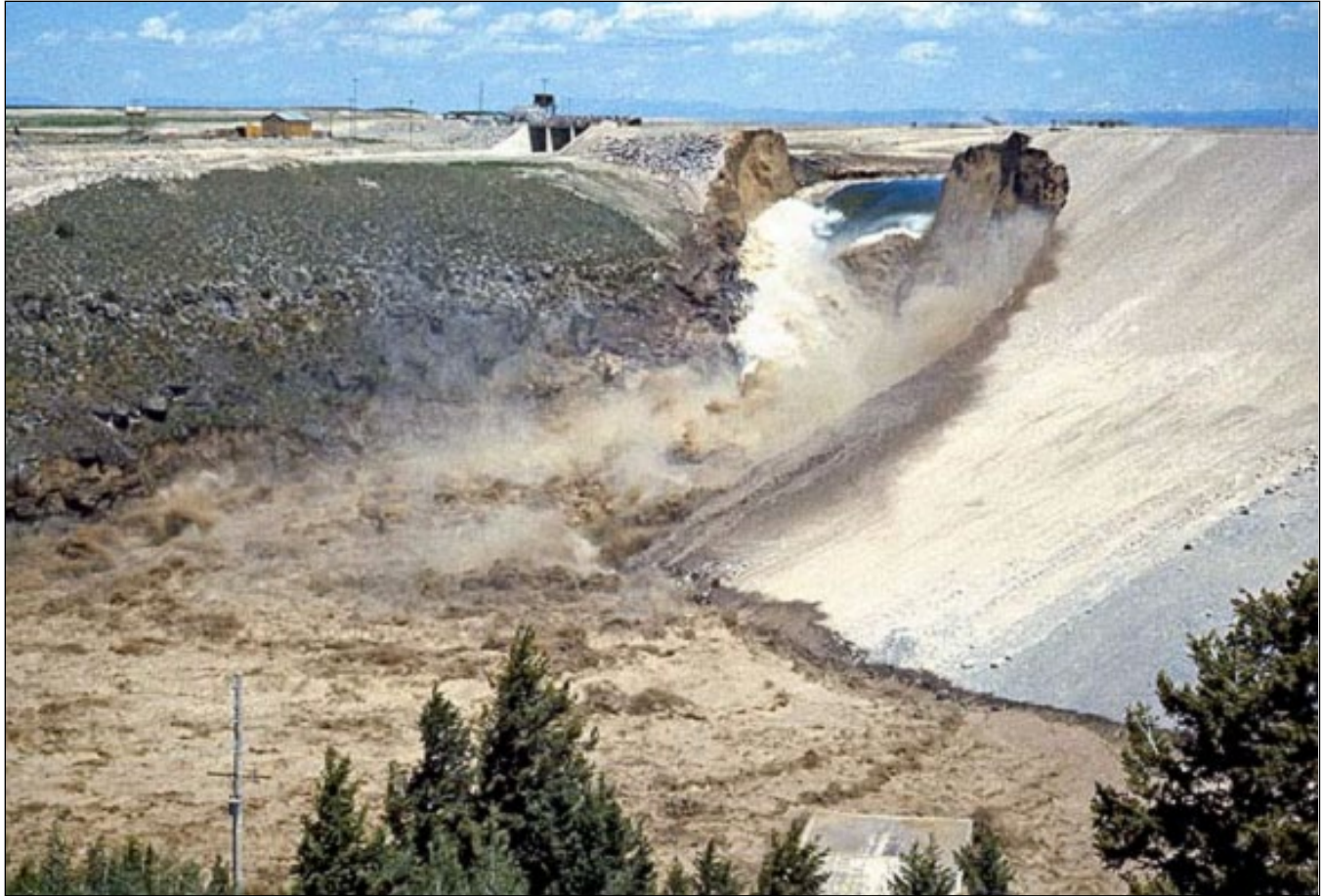
Figure 10-1. Teton Dam Failure, 1976
