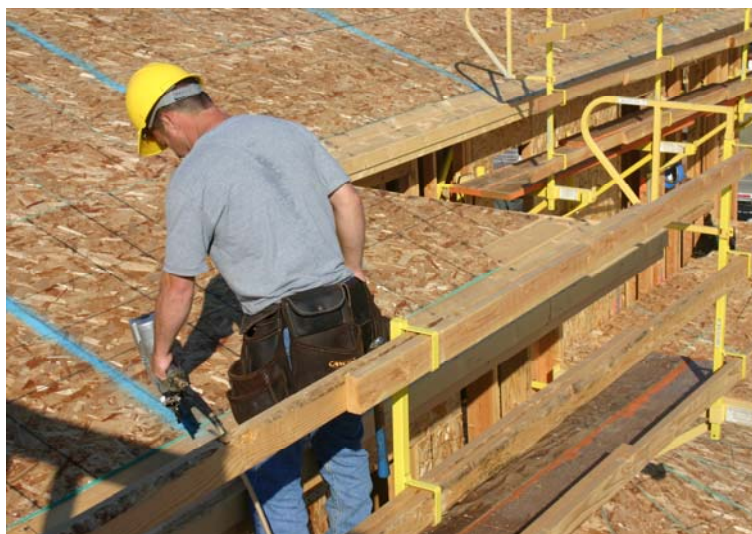
Figure 8 – A worker sheathing a roof from a bracket scaffold.
