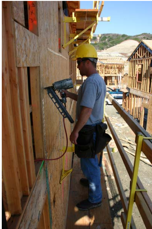
Figure 29 – A worker sheathing walls from an exterior bracket scaffold.
