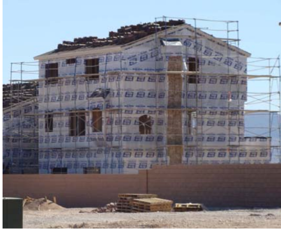
Figure 28 - Welded end frame scaffold.
